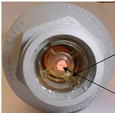
1. To set the flow meter on the Water Block use the white key provided to move the arrow to number 1 on the inside of the rim. This will limit the flow to 4.5 ltr. If the arrow points to 2, the flow will be limited to 9 ltr. Each incremental number raises the flow limit by 4.5 litres.
